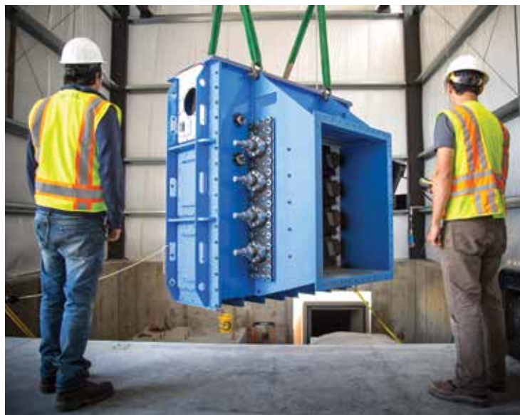
Natel's hydroEngine™ generates power at drops between 6 and 60 feet in height.
