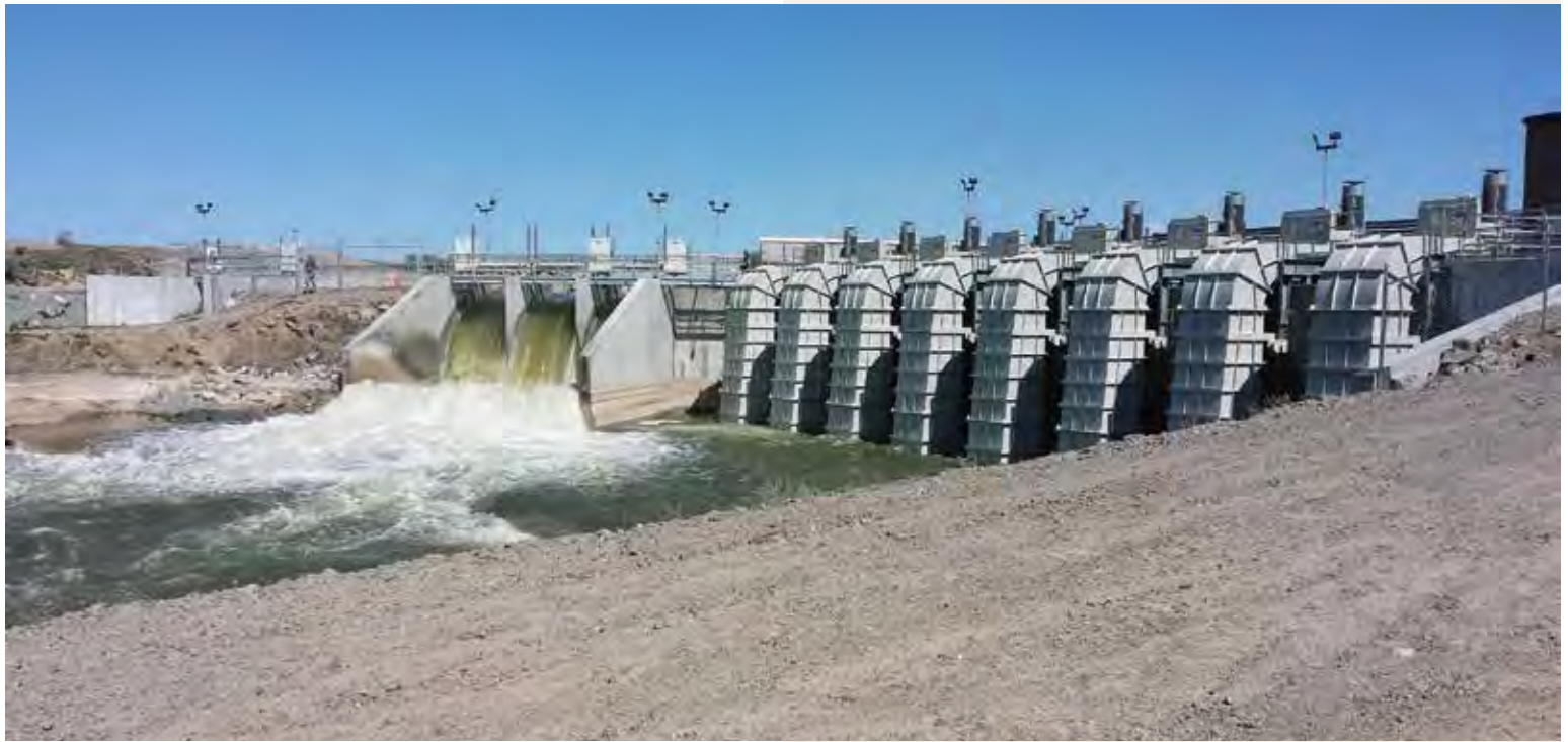
Downstream side of the new facility.
